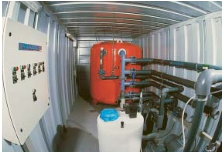
EUROWATER pressure filter built into a container.
